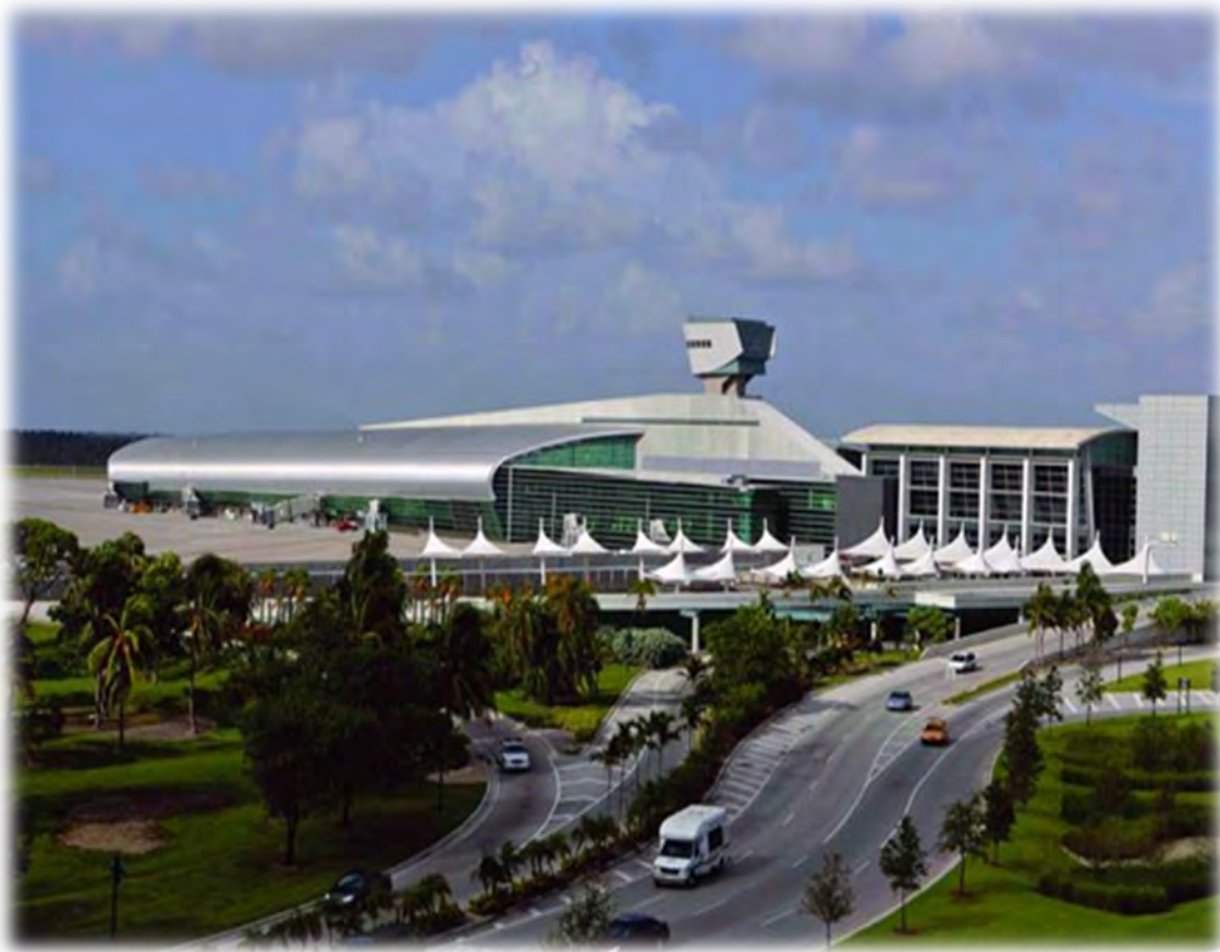
Miami International Airport Concourse J
